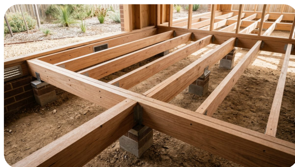
Repaired, not patched — proper structural restoration.
